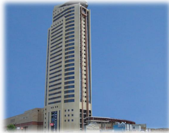
Palladium Tower with RF Repeaters
