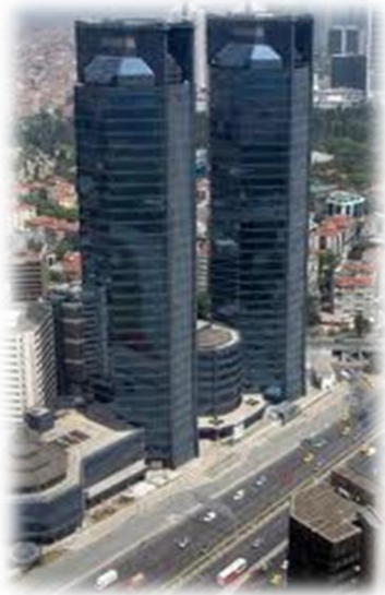
TAT Towers with RF Repeaters
